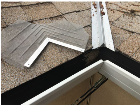
Step 1: Prepare area, trim edges to fit
