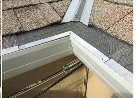
Step 3: Install Gutter Guard on both sides
