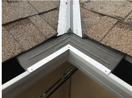
Step 2: Under Shingle or Fascia Mount
